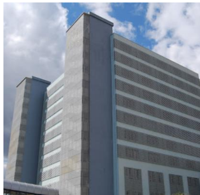
Figure 7. Emergency Clinical Hospital "Bagdasar-Arseni", Bucharest.
